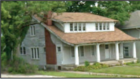
This is what the house looked like before UM Men repaired, repainted and renovated it.
